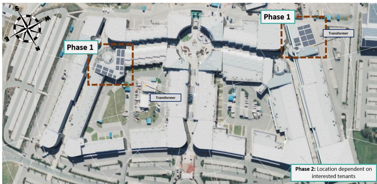
Figure 11: 150 kWp (phase 1) South-facing solar PV installations on existing roof
